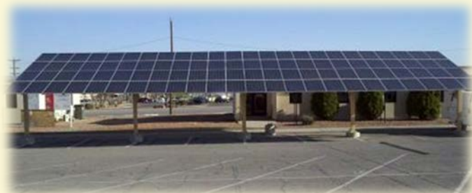
(Photo by USACE SWD)
